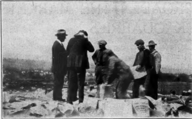
Loading Well Drill Shot, Top of Number 3 Quarry
